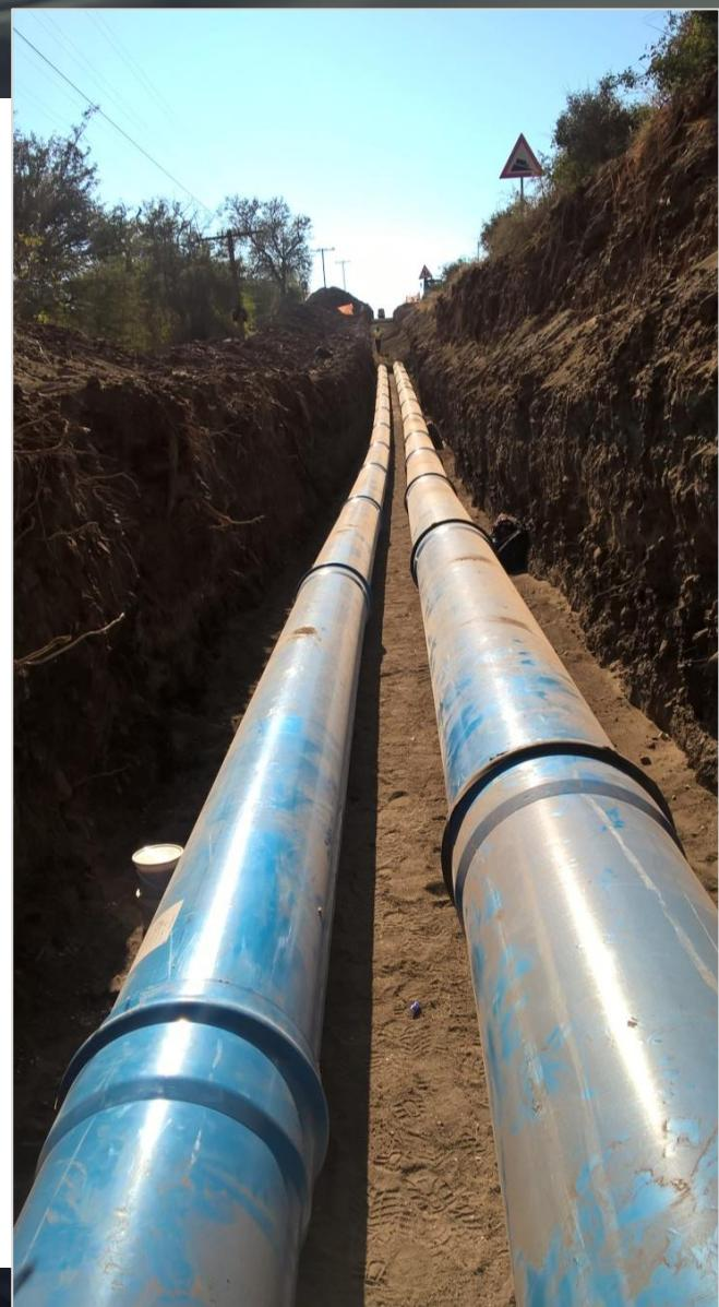
water system, optimisation of pipe diameters, velocities and internal pressures to achieve the desired flows. Construction drawings for the bulk pipelines and branches were produced including details of isolation, scour and air valve chambers; bulk water meters and inline booster pump stations.
